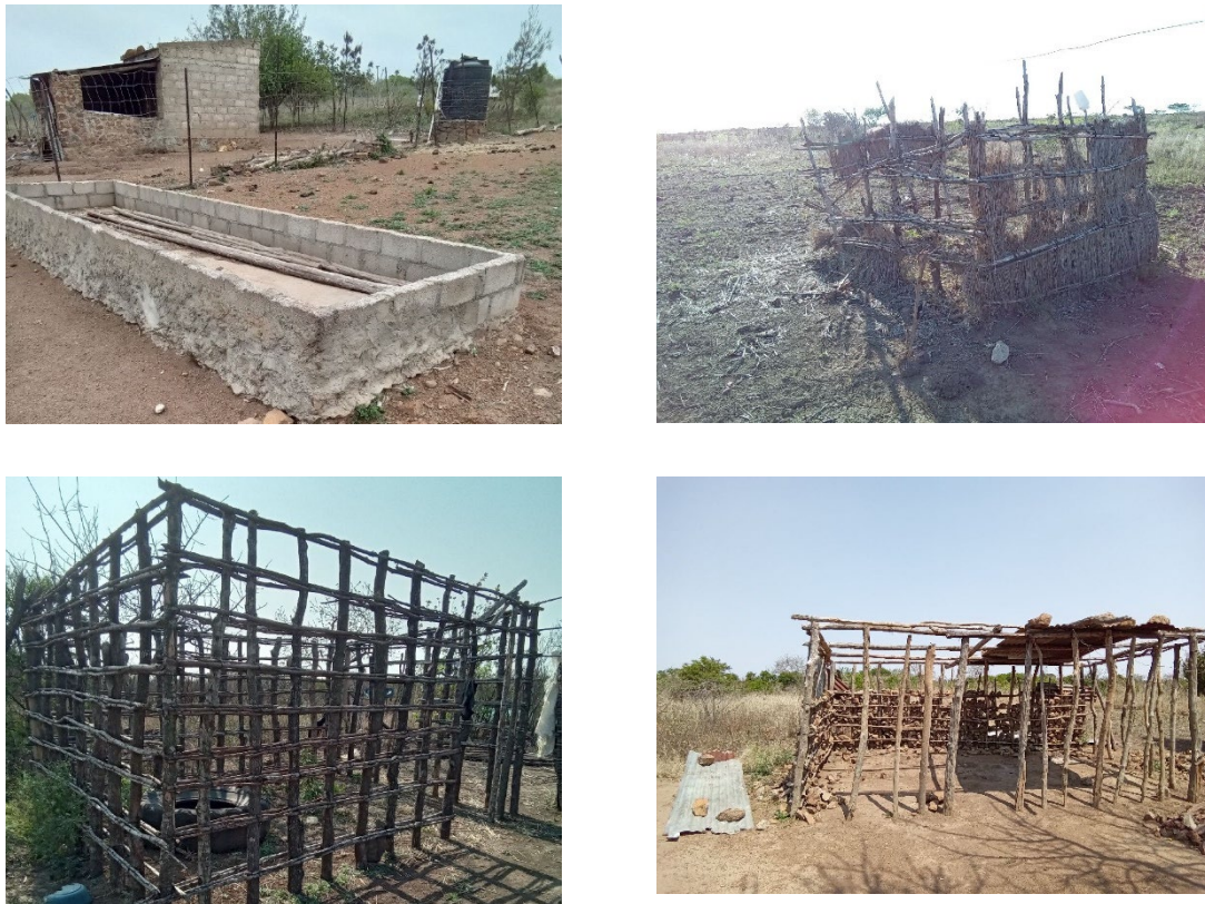
Figure 6-3 – Structures Under Construction
